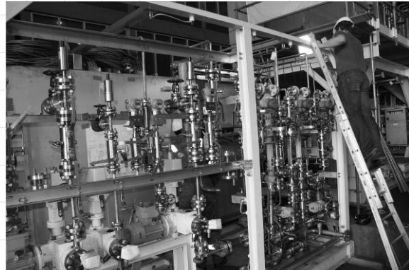
Methanol injection skid developed in cooperation with Frames Energy Systems BV
